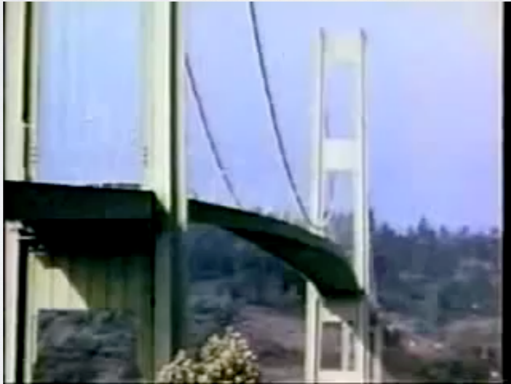
Tacoma Narrows Bridge collapse (1940), www.youtube.com/watch?v=3mclp9QmCGs
