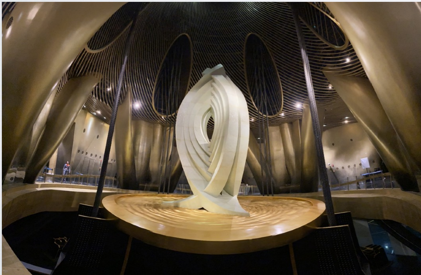
Damper in Shanghai Tower (1000t, using oil damper + eddy currents), Wiki commons
