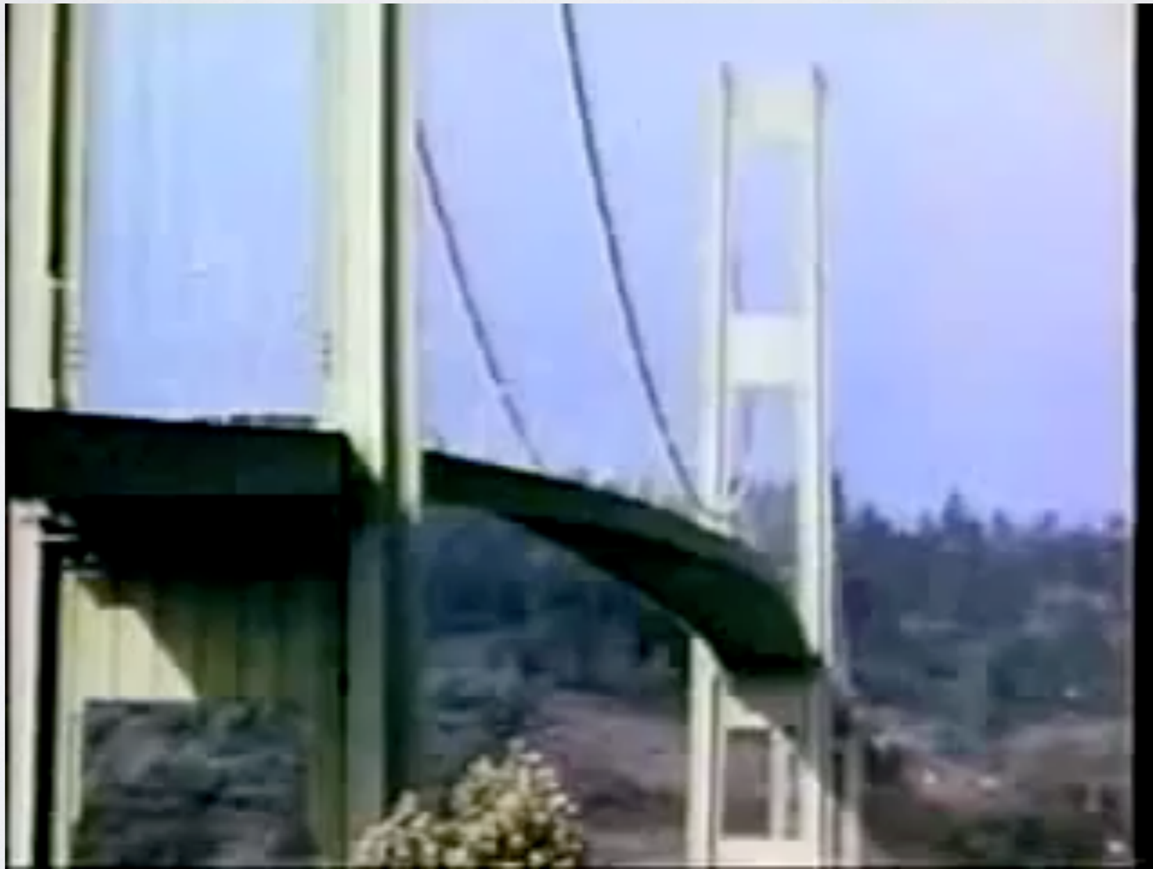
Tacoma Narrows Bridge collapse (1940), www.youtube.com/watch?v=3mclp9QmCGs
